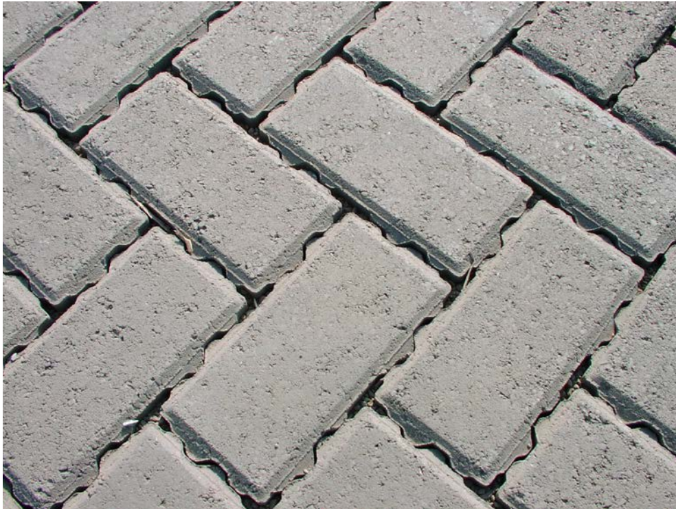
Figure 1. Priora Permeable pavers installed in herringbone pattern
